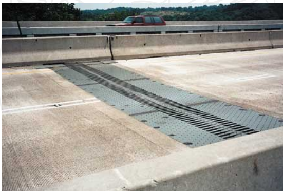
1. Figure: Expansion joint
